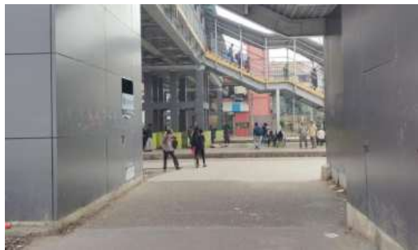
Major facelift: Officials say 90% of the construction work for a new booking office at the station has been completed. T. ARVIND
